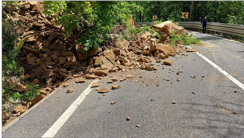
Figure 35. Rockfall in the Lepsa area, on the national road DN 2D.
