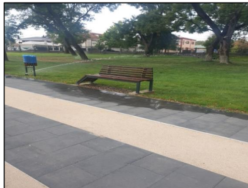
Figure 9. Malfunctioning irrigation system
